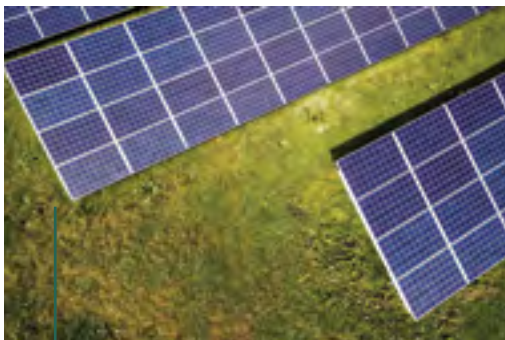
Panneaux solaires - Source : Andreas Gückhorn on Unsplash
